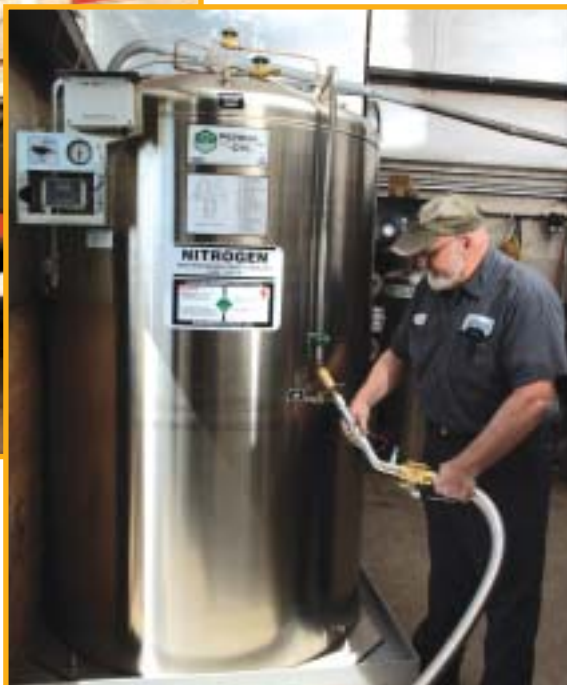
Airgas driver, Kenneth Alexander, refills Cutting Edge Laser's microbulk tank (left) and adjusts the VHP Perma-Cyl below. The truck maintains pressures between 420-450 PSI during refills, helping to reduce downtime.
