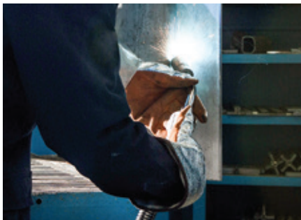
All position welding
