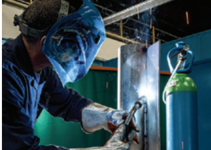
MIG welding of carbon steel
