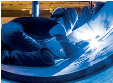
TIG welding of stainless steel
