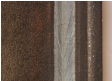
Clean weld surface
